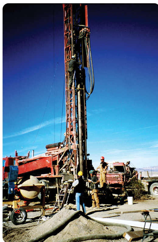
Lowering instrument cables and gas-sampling tubes into a 110-m-deep unsaturated zone borehole. Photo courtesy of Brian Andraski.
