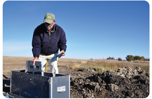
Dan Jaynes of USDA-ARS inserts panels into a water control structure that diverts water from field tile into tile that runs parallel to the stream, which then flows into the saturated riparian buffer. Photo by Lynn Betts, USDA-NRCS.
