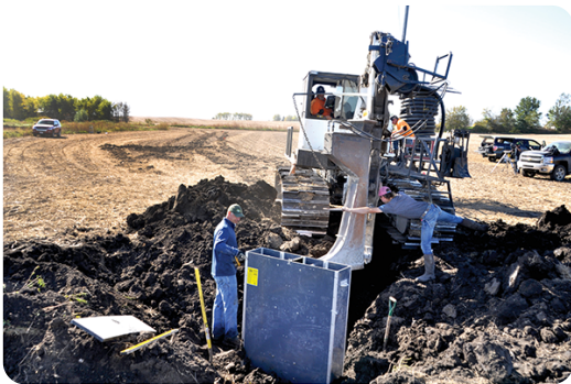
A water control structure (foreground) is placed into the field to divert water from field tile to perforated tile running parallel to the stream, saturating the buffer. Photo by Lynn Betts, USDA-NRCS.
