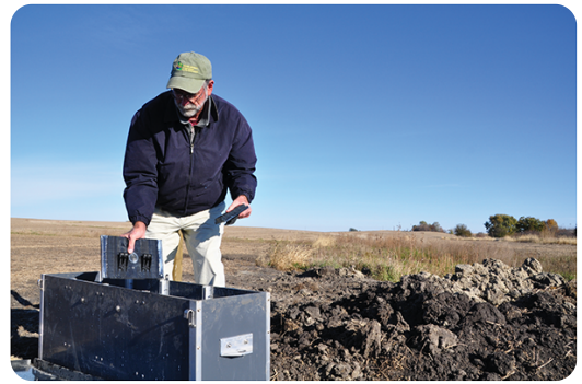
Dan Jaynes of USDA-ARS inserts panels into a water control structure that diverts water from field tile into tile that runs parallel to the stream, which then flows into the saturated riparian buffer. Photo by Lynn Betts, USDA-NRCS.
